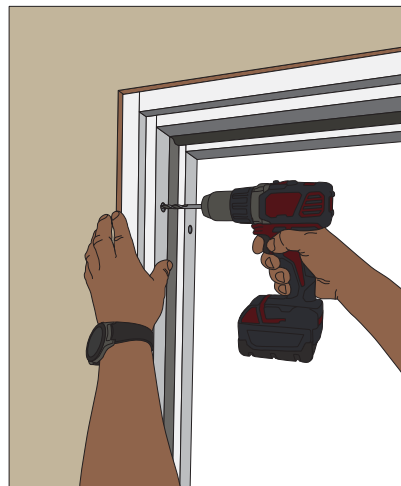
STEP 11. Fix the lock side of the door frame to the wall (drill the wall through the adjustable hole or installation bolt points in the vertical part of the door frame).
