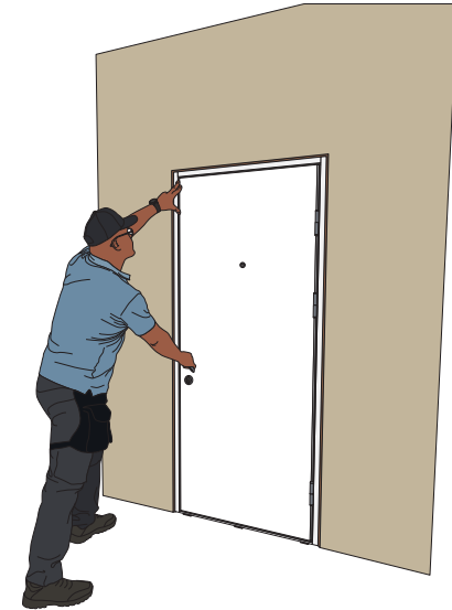
STEP 9. Check the closing function and gap seals.
