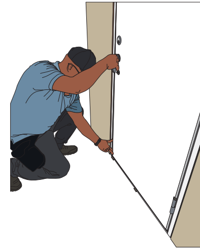
STEP 15. When both sides of the door frame are fixed in the wall opening, put the gap appropriate pads under the middle and lock side of threshold.
