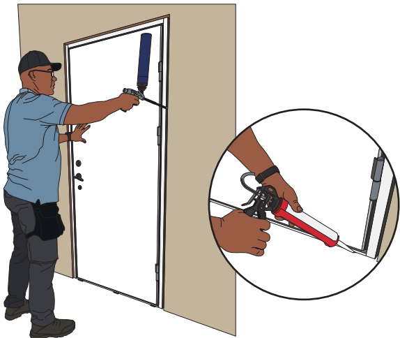
STEP 16. Depending on the product specifications, the gaps between the wall and the door frame may be sealed using the following materials: Penosil Premium Fire Rated B1 fire resistant polyurethane foam, Paroc Extra mineral wool.
